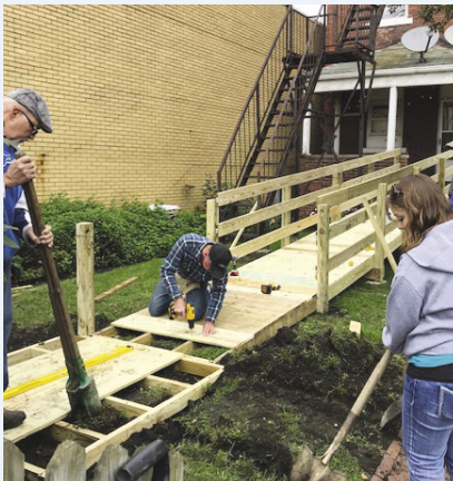
Ramps of Hope volunteers install a new ramp.
